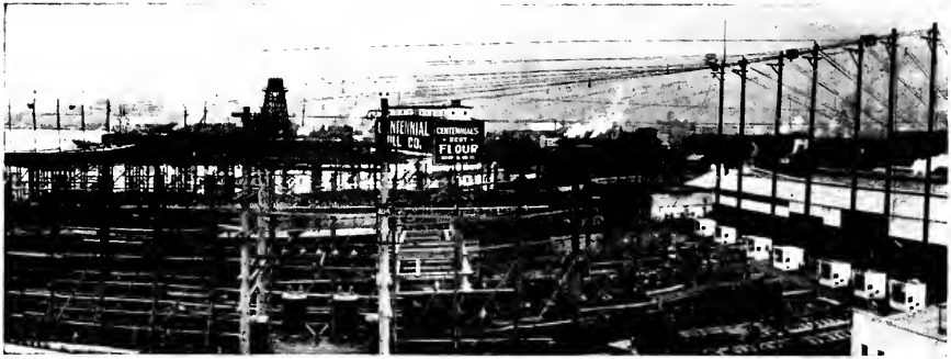
This picture illustrates the trolley system for handling material over the building ways.
